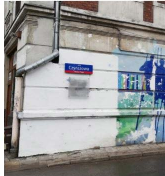
Fragment after filling cavities. Photo S. Woropaj
