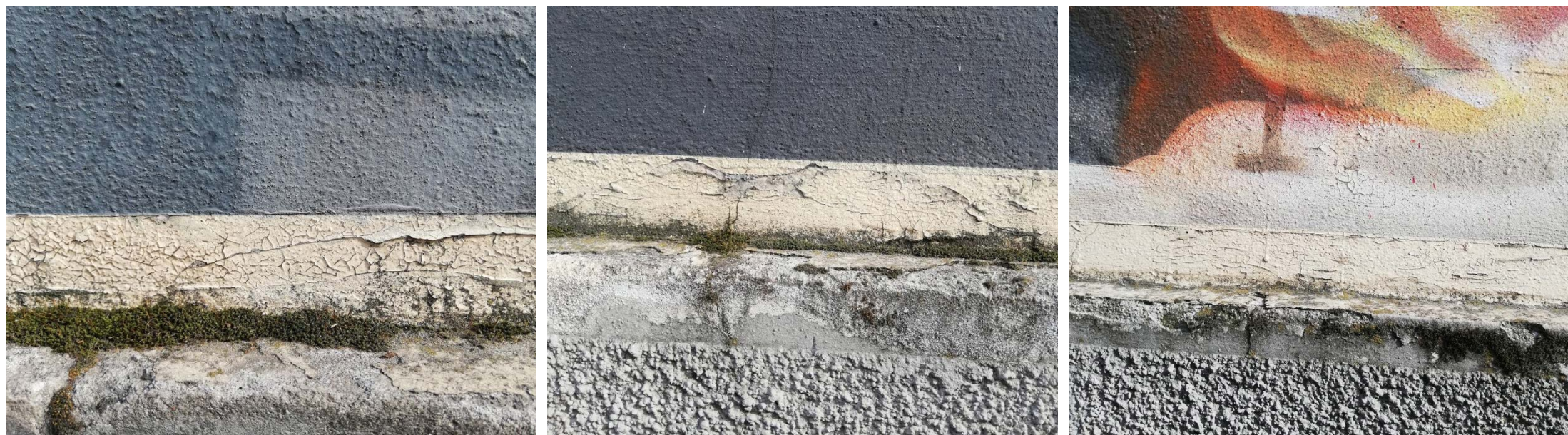
Close-up images of the protrusion localized along the edge between the mural and the lower concrete socle.
