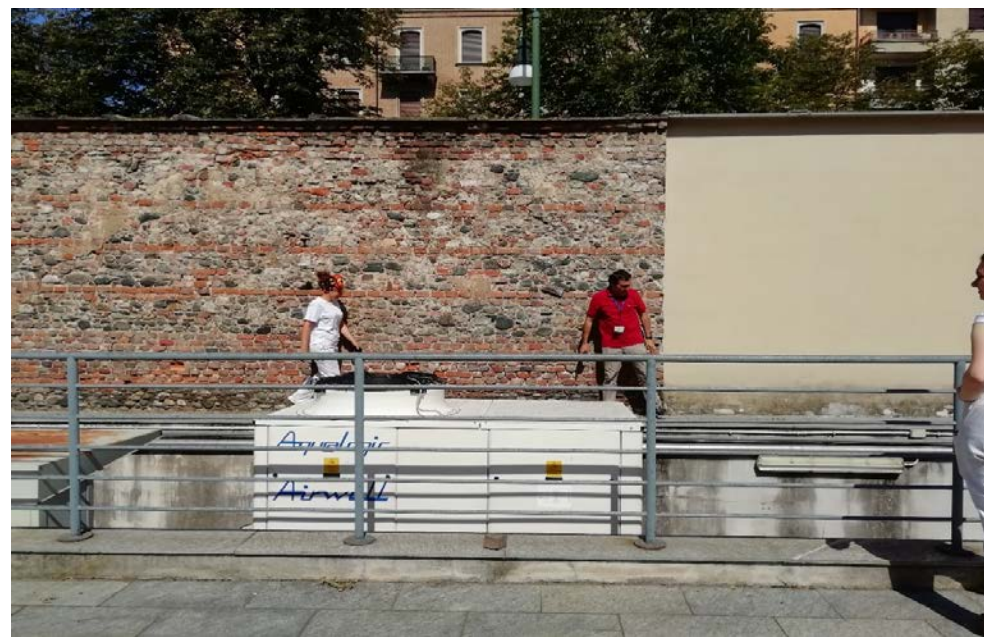
Photo of the back side of the wall showing the ancient brick-and-stone structure and the modern light yellow painted cladding.
